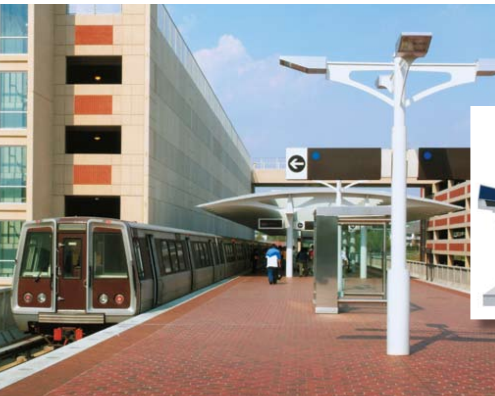
The precast concrete boarding platform, the first of its kind in the Washington, D.C., Metro system, is flanked by two parking structures with all-precast concrete structural systems at the Largo Town Center station.
